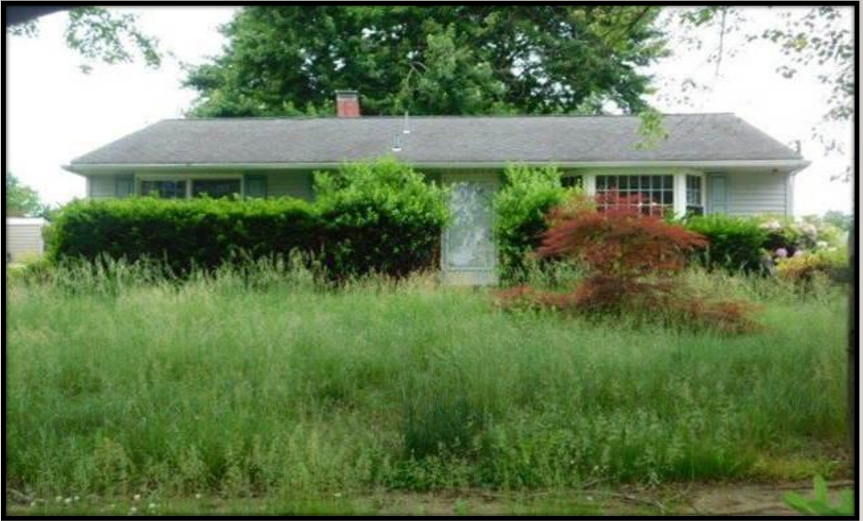
Property Maintenance Issues (Exterior)
